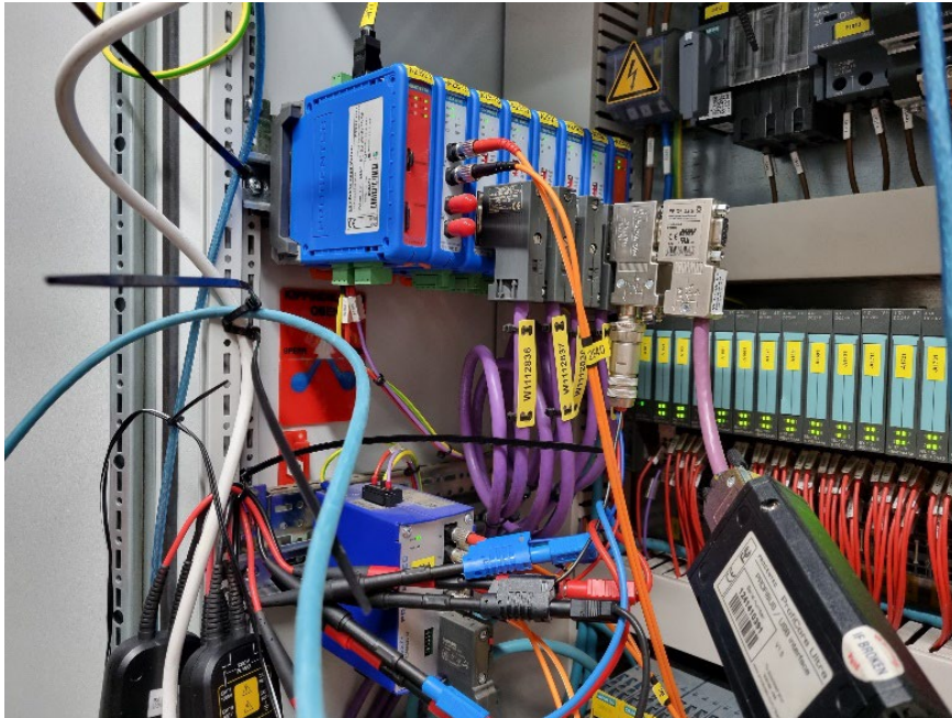
Figure 143: Detail of the PROFIBUS devices (ComBricks) inside the cabinet
