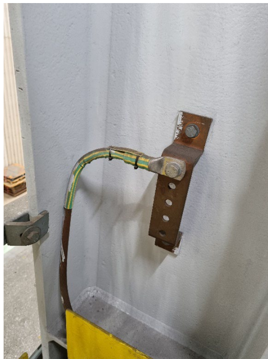
Figure 138: PE connection to the building's earthing
