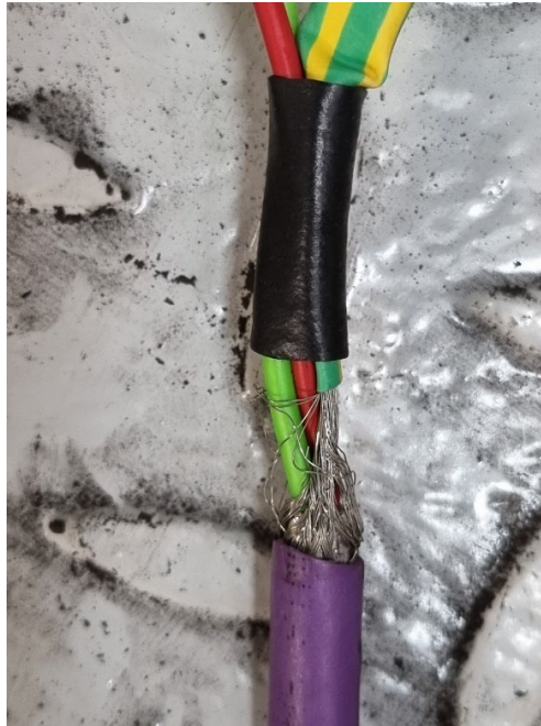
Figure 146: Detail of the PROFIBUS cable (1)
