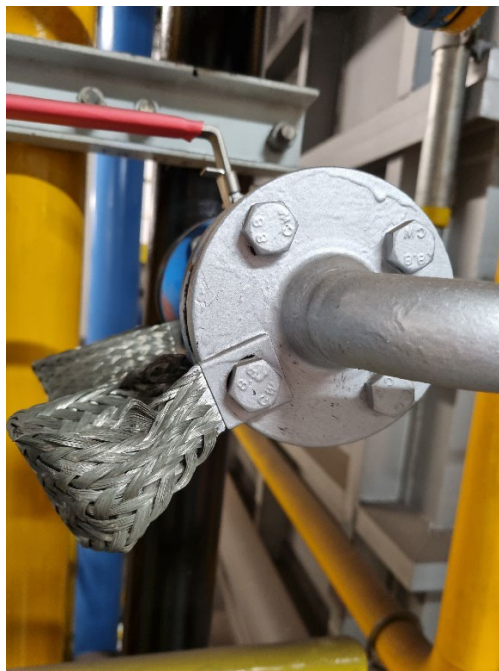
Figure 136: Litz wires on the gas installation (1)
