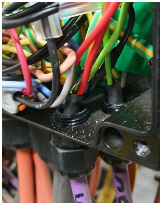
Figure 145: PROFIBUS cables entering the Dungs cabinet
