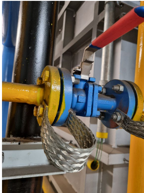
Figure 137: Litz wires on the gas installation (2)
