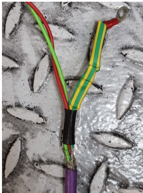
Figure 147: Detail of the PROFIBUS cable (2)
