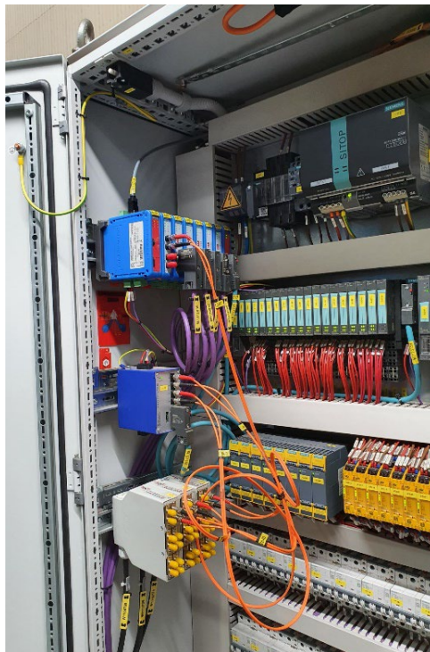
Figure 142: PROFIBUS devices (ComBricks) inside the cabinet
